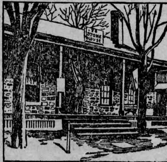
"ANDRE'S PRISON." (Historic Building Which New Yorkers Want Preserved.)
