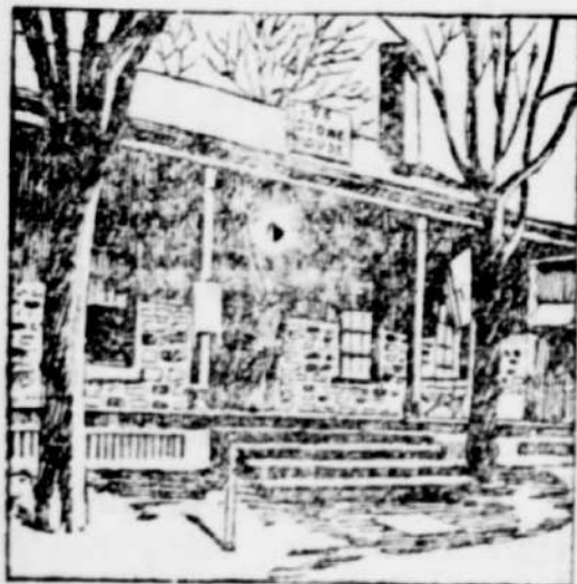
"ANDRE'S PRISON." (Historic Building Which New Yorkers Want Preserved.)
